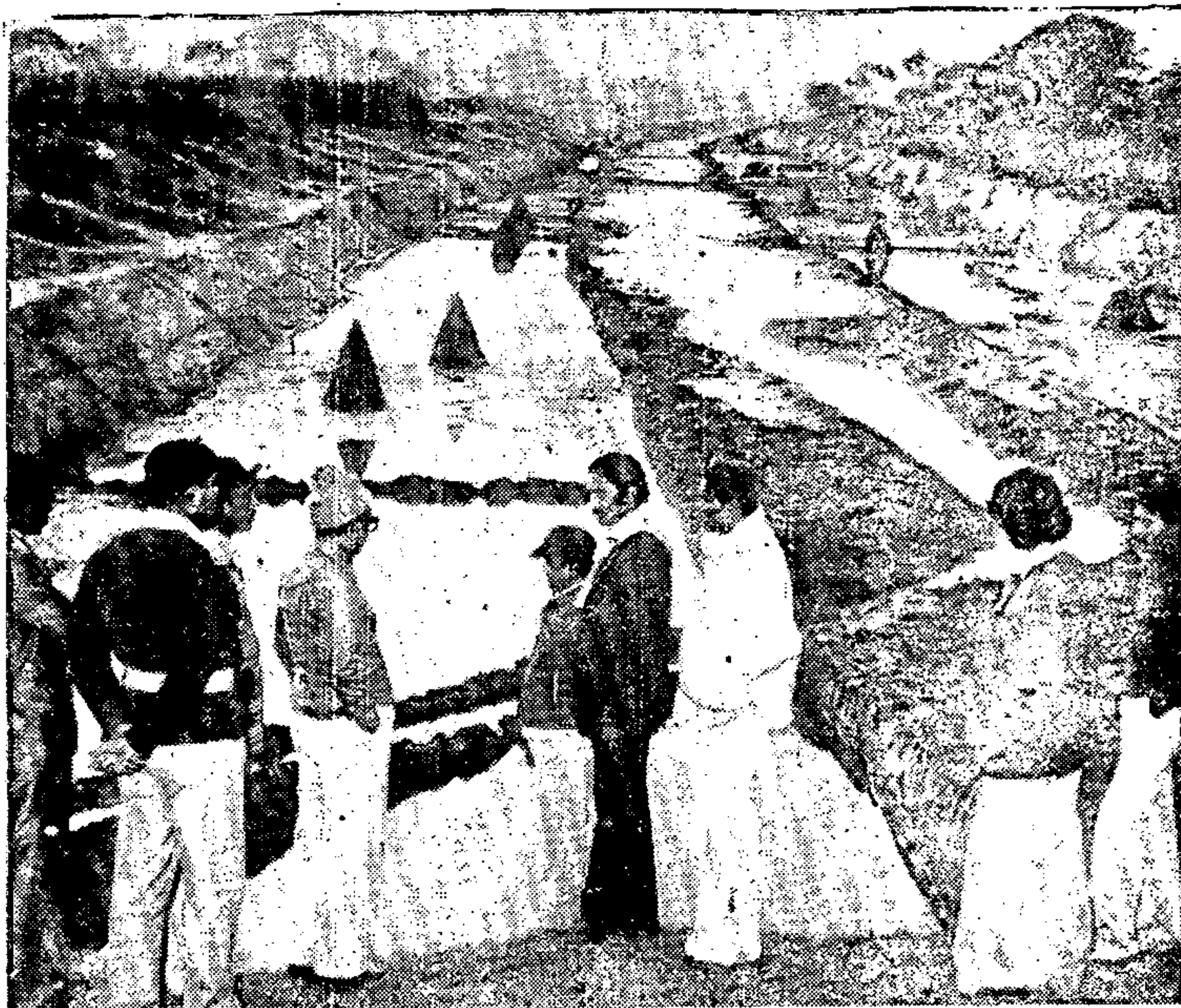
Prime Minister Shah Azizur Rahman inspecting the progress in Hisna river re-excavation project at Daulatpur, Kushtia on Saturday. President Ziaur Rahman inaugurated the project on December 14 last. —Photo: FIU
