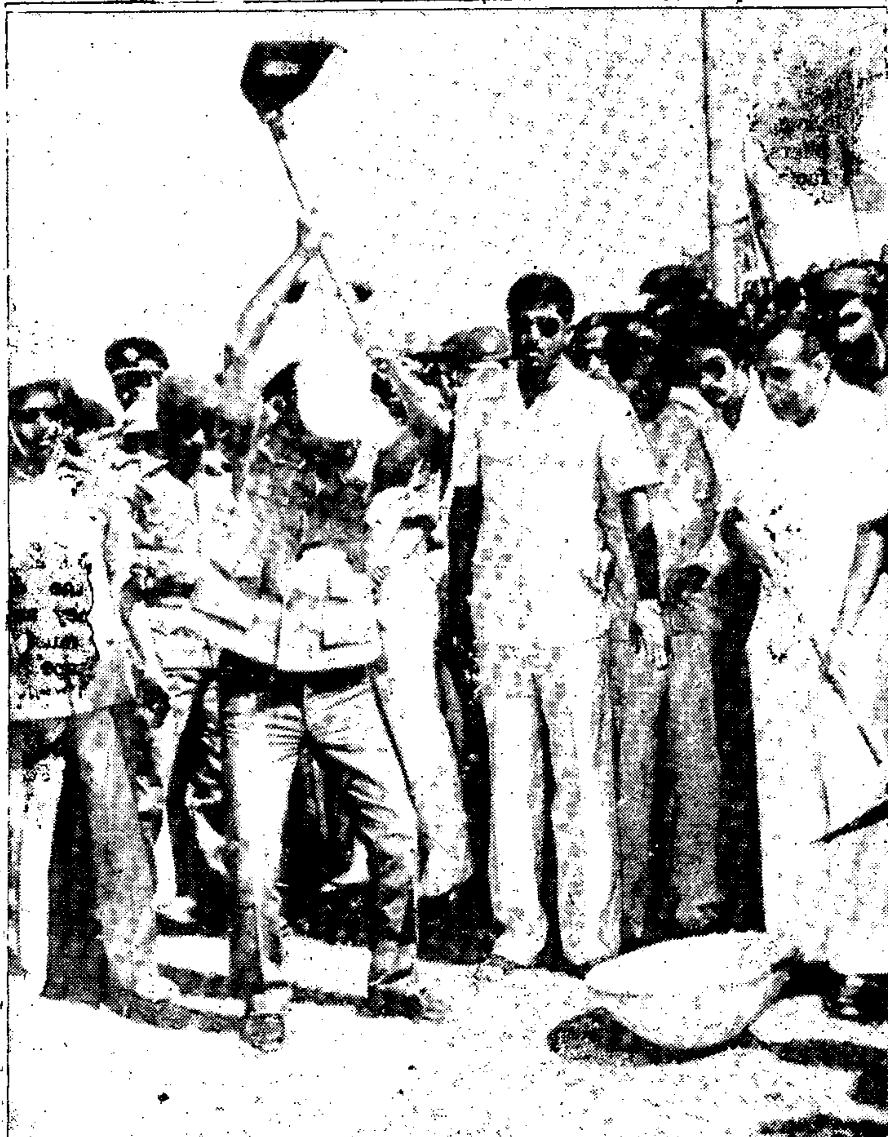
President Ziaur Rahman inaugurated the excavation work of a canal beside Gohall-Chandibar Road in Bogra on Saturday. — Photo PID.
